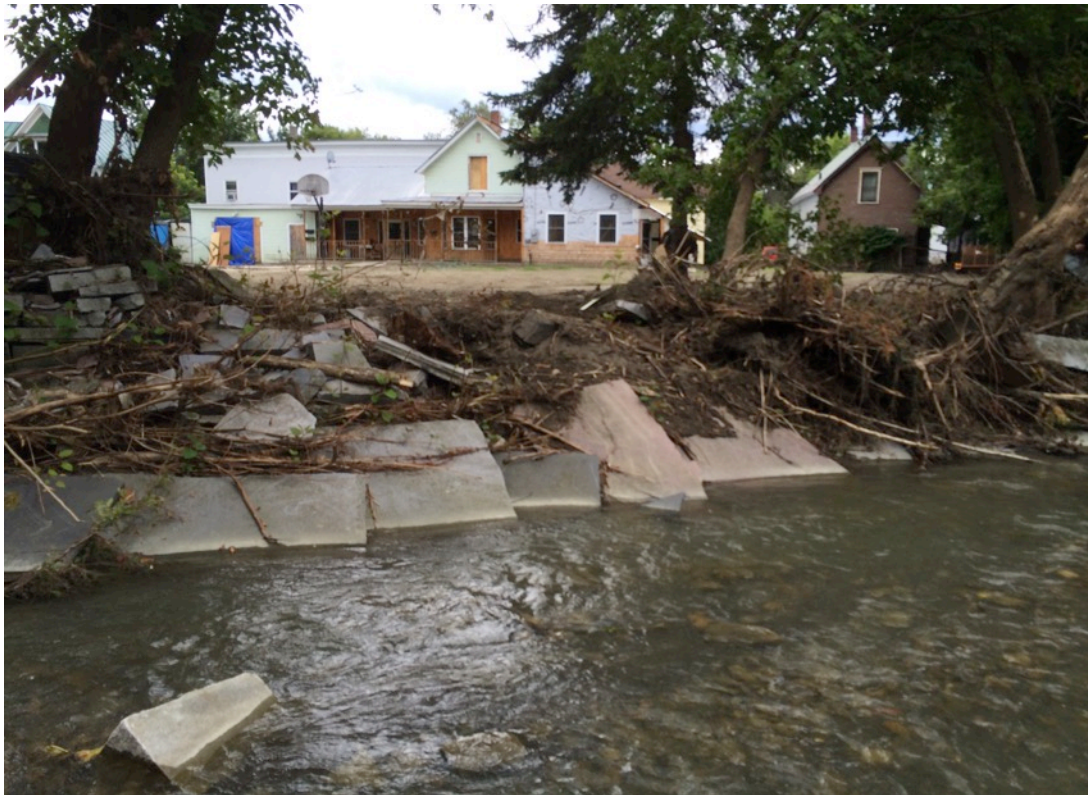
Left floodplain restoration area
