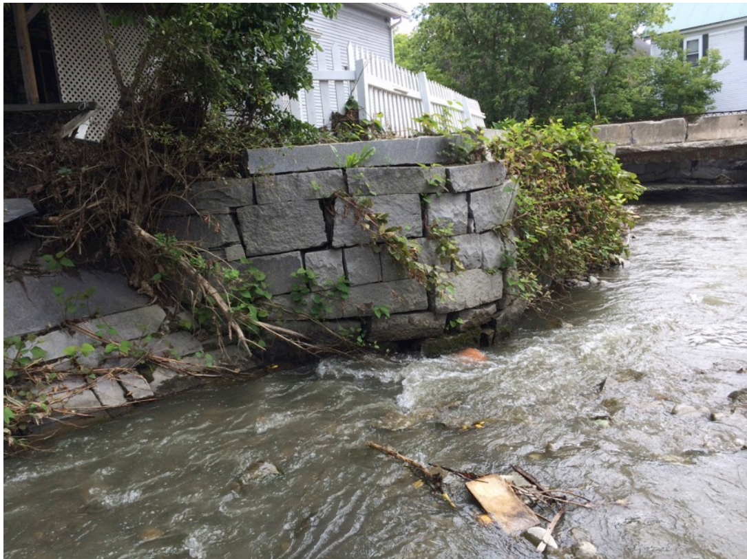
Severe channel constriction at Harrington Ave. bridge
