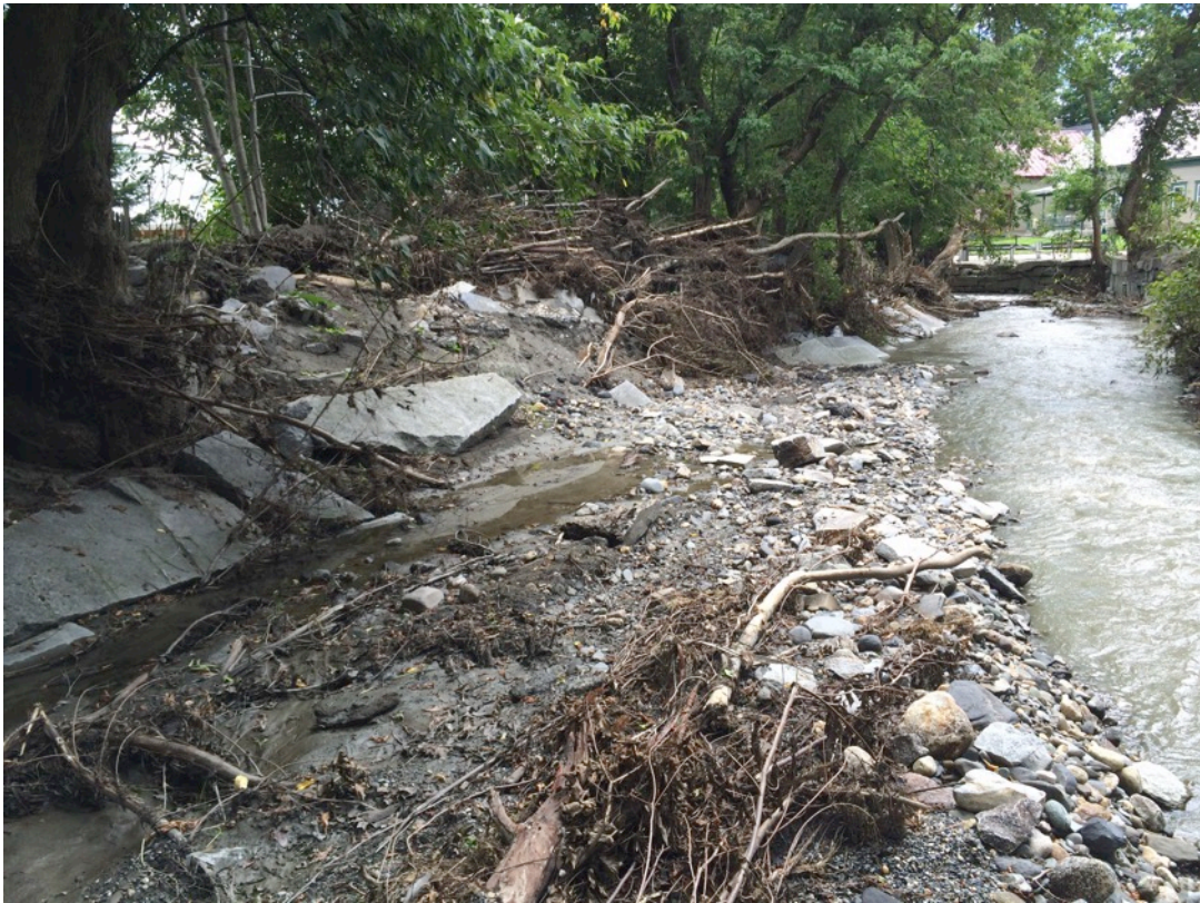
Bank restoration area just upstream of Harrington Ave.
