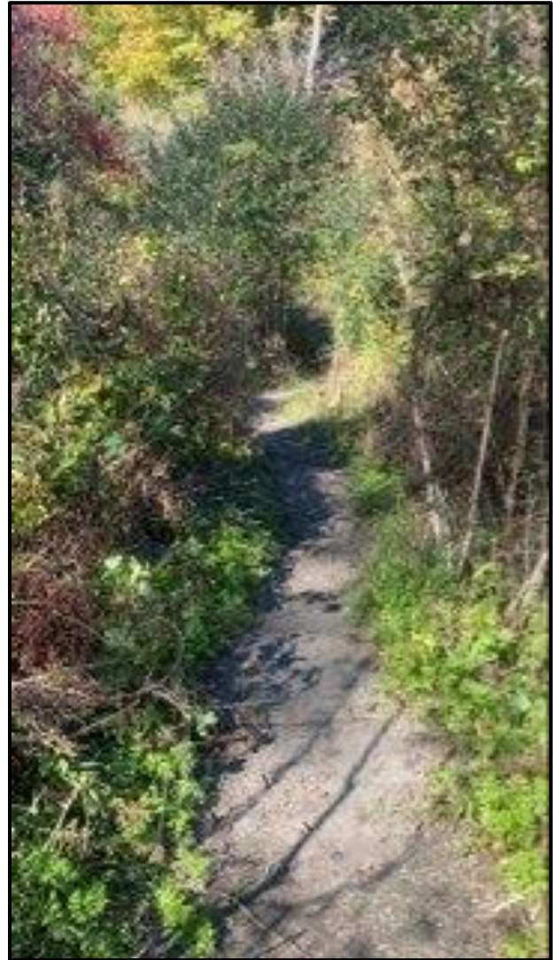
ABOVE: PICTURE OF THE IMPROVED TREAD THAT IS BRUSHED OUT AND LEVELED WITH CONSISTENT OUTSLOPE FOR IMPROVED DRAINAGE
