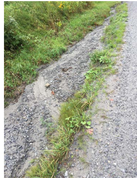
Figure C13. A section of Middle Road where roadside ditches are filled with sediment.
