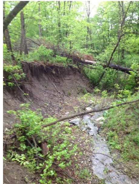
Figure C9. Stormwater that drains to the pictured gully from both the Health Center's detention pond outlet and from an unmanaged stormwater outfall. Significant erosion has occurred.
