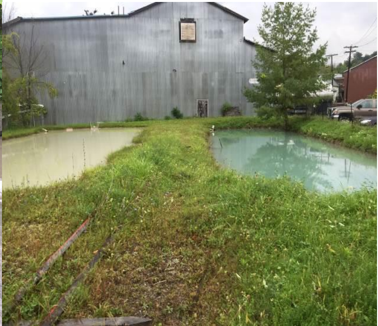
Granite processing waste pit within the riparian area on Boynton St.
