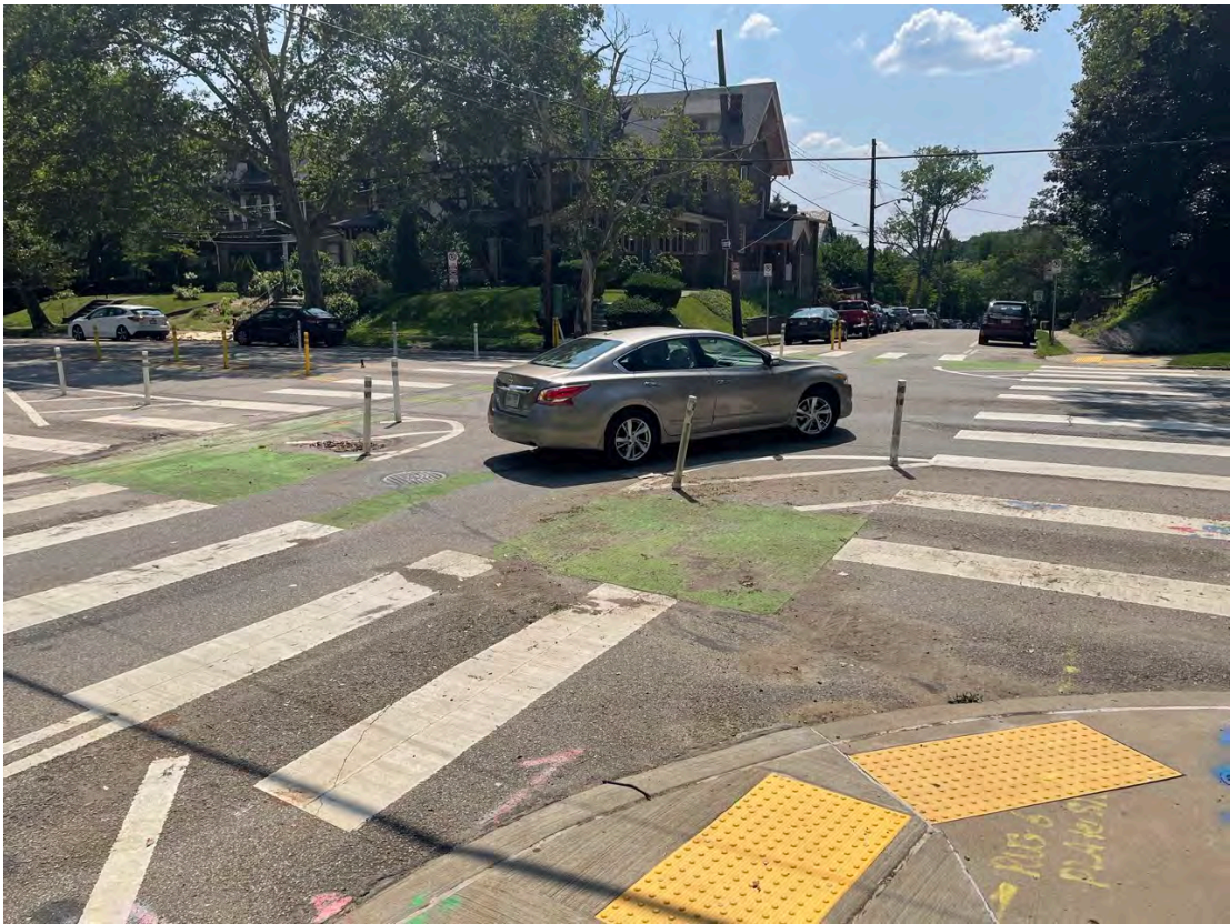
Similar treatment observed in the field (with bike lanes)
